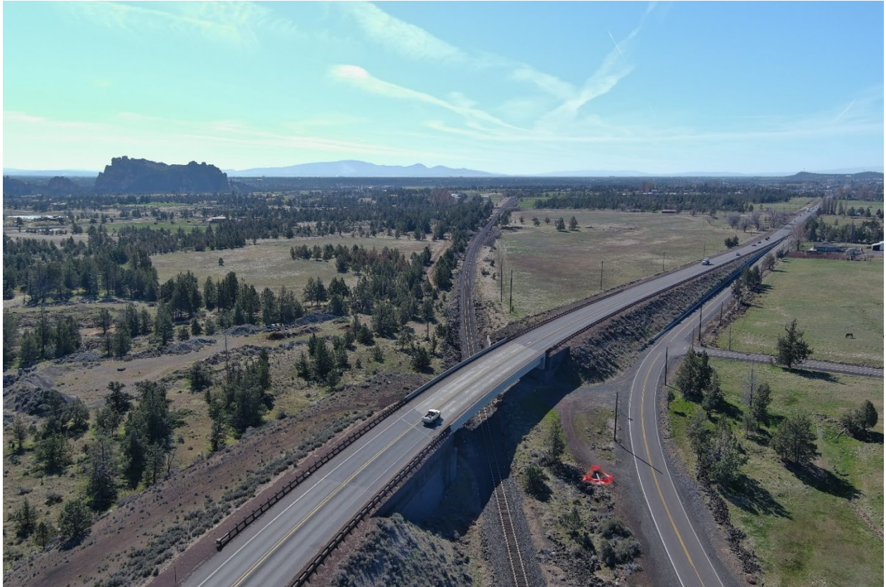
Figure 6.9 US 97 Railroad overcrossing
